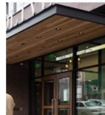
9 Metal canopy with wood soffit, wood doors, & aluminum storefront
