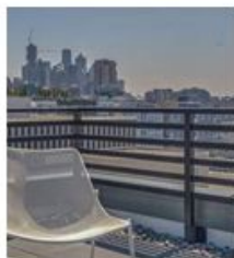
3 Metal railing & concrete pavers
